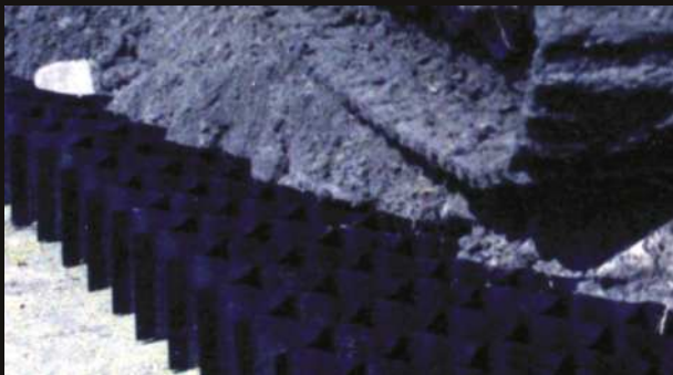
TEMPORARY SERVICE ROAD THROUGH FLY-ASH SETTLING BASIN
