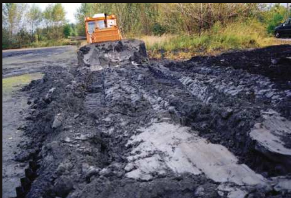
TEMPORARY SERVICE ROAD THROUGH FLY-ASH SETTLING BASIN
